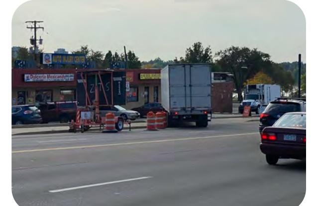
Delivery truck utilizing driveway north of 25th Avenue
