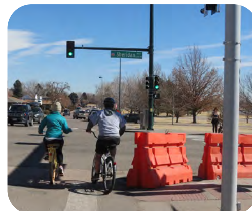
Traffic calming elements in place at 25th Avenue
