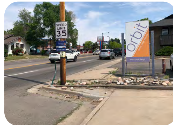
Attached sidewalk with obstruction south of 26th Avenue
