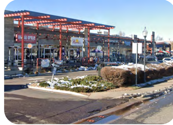
Off-street parking for businesses north of 20th Avenue
