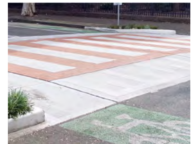
Raised pedestrian crossing
