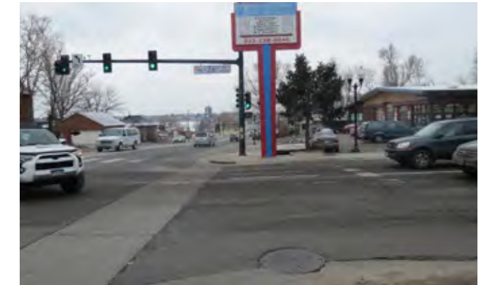
26th Avenue Intersection - crash hotspot
