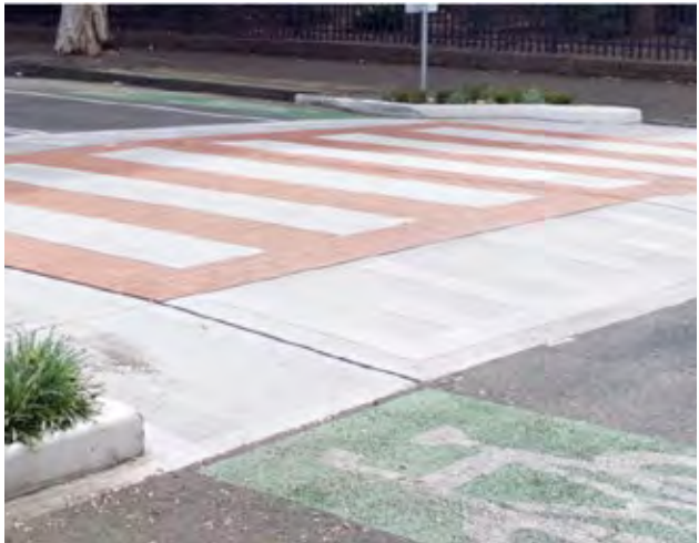
Raised pedestrian crossing
