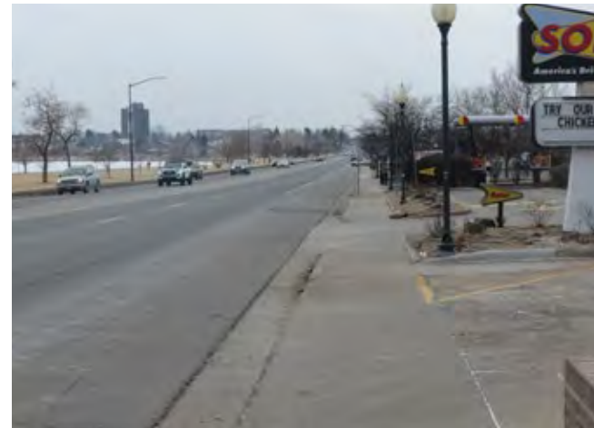
Narrow sidewalk next to travel lanes
