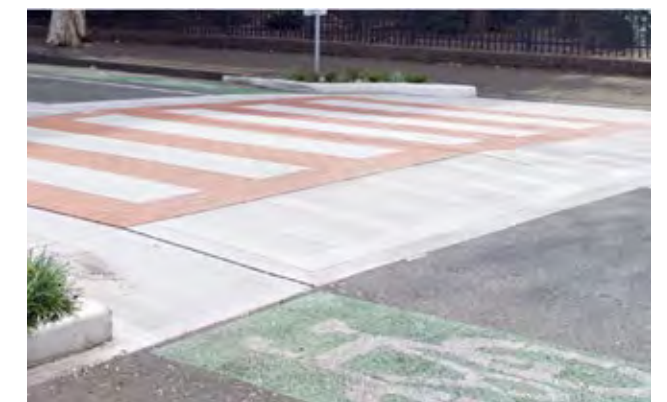
Raised pedestrian crossing
