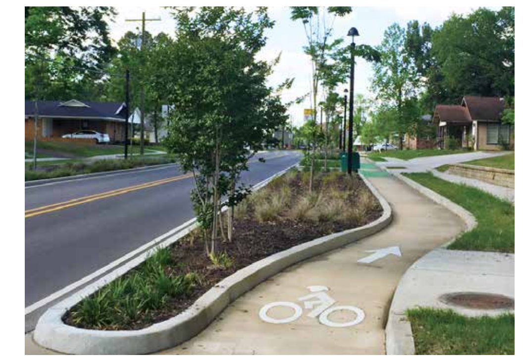
Median protected bike lane
