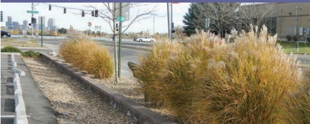
Low Impact Design Storm Water Swale (20th Avenue & Ames Street)
