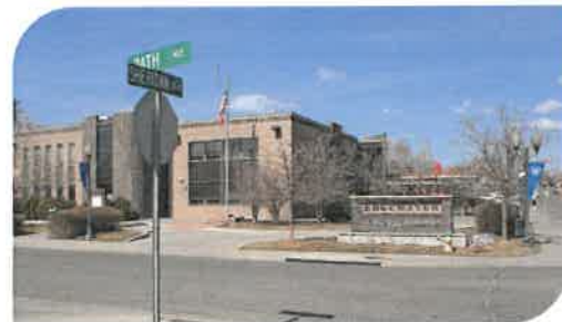
Old Edgewater Municipal Building
