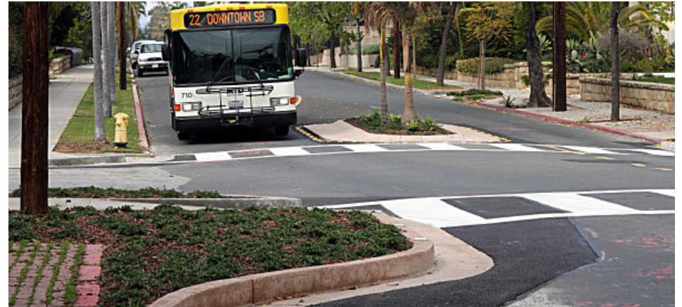
Above: A large vehicle being deflected through a neighborhood Intersection Chicane | Santa Barbara, CA
