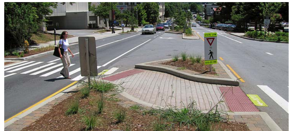
Above: Pedestrian crossing island | Charlotte, NC
