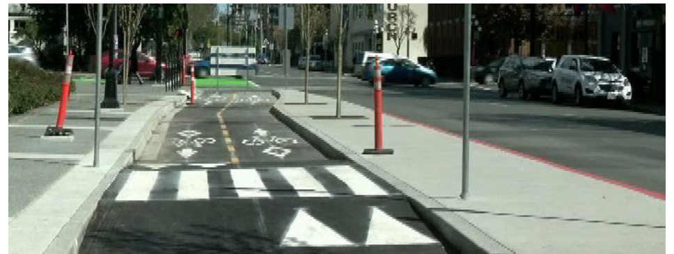
Below: Raised table crossing and bus-bulb | Victoria, BC
